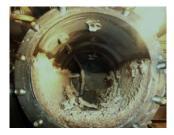
In some cases, a majority of the scale are removed manually but in other cases, the nature of the minerals may be resistant. The boiler and all tubing are soaked in an agent such as citric or phosphoric acid. The acid is left for a period of time, then removed and the boiler and tubing are flushed.
